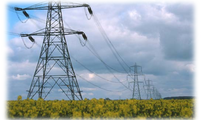
Transmission Line Project
