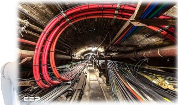
Underground Cable Project
